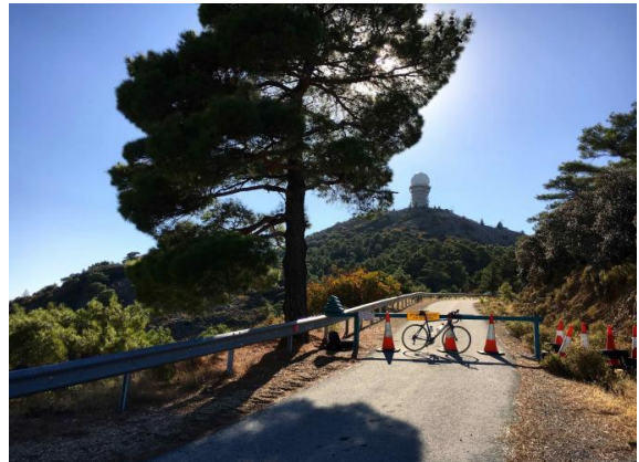
Radar on Mount Kionia
