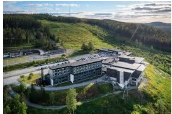
The Hallstaberget dominates the area
