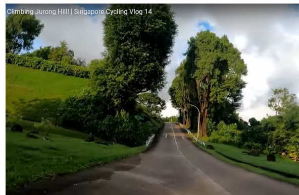
The final ramp.
